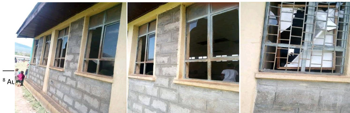
Figure 1: One of conflict-affected schools (Buno Primary School, Chelelektu Woreda)
