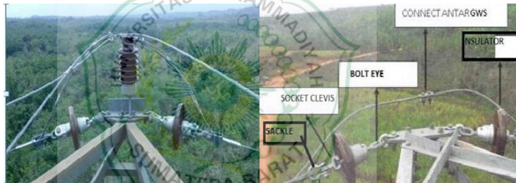
Gambar 3.5. Rangkaian Insulator Tension
