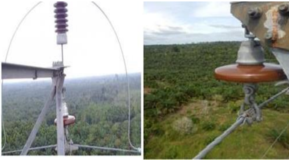
Gambar 3.6. Rangkaian Insulator Suspension
