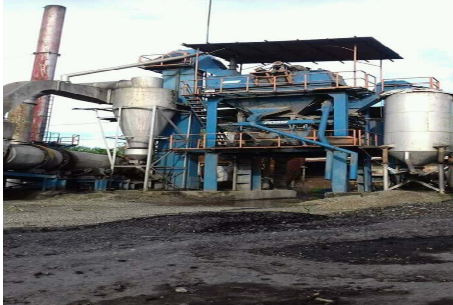
Gambar 2.5 Asphalt Mixing Plant (AMP)
