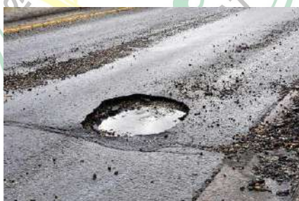
Gambar 2.8 Lubang ( Photoles )
