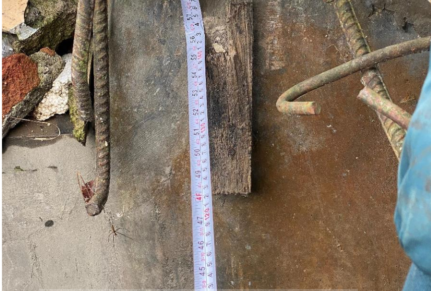
Pengukuran Drainase Eksisting Lebar 1,5m STA 0 + 000
