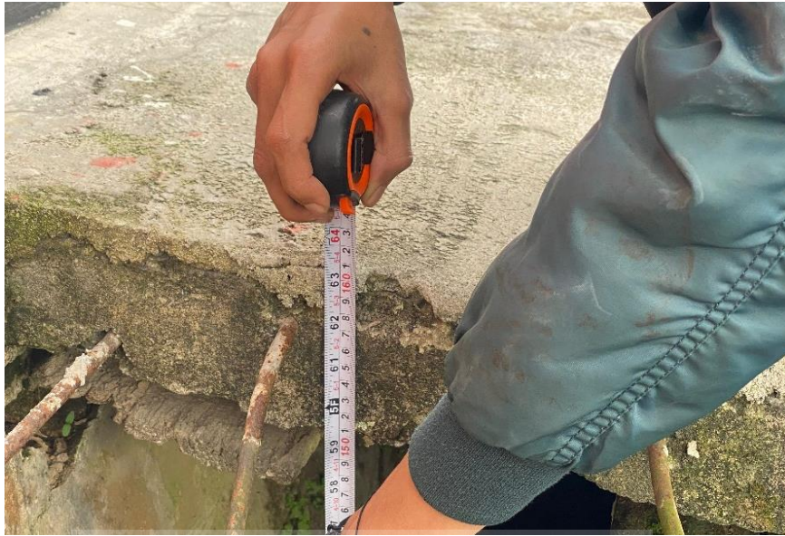
Pengukuran Kedalaman Drainase Eksisting Kedalaman 1,3m STA 0 + 800
