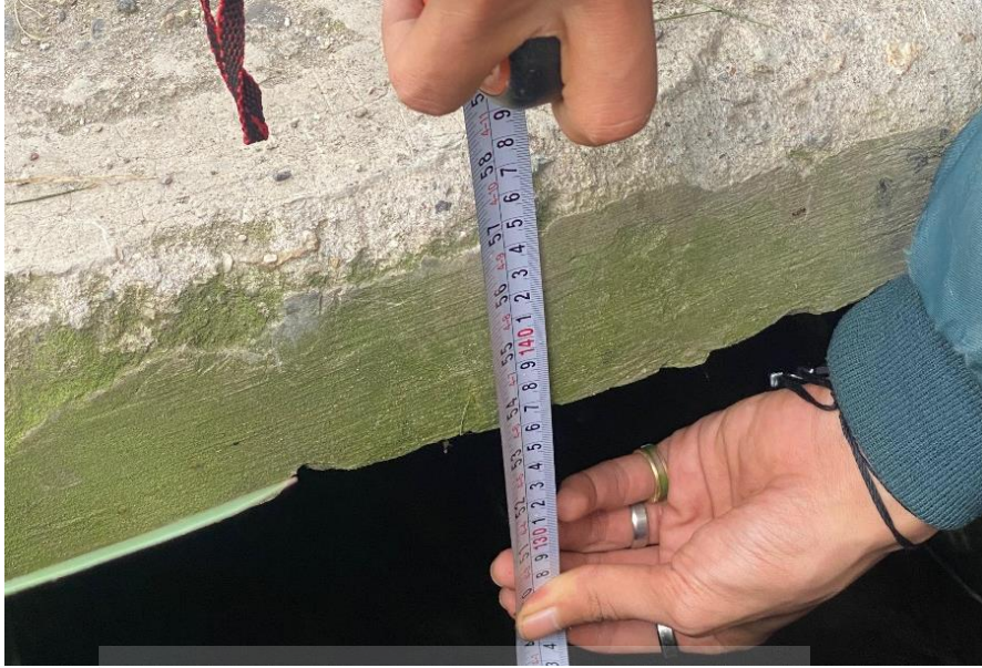
Pengukuran Saluran Drainase Eksisting Kedalaman 1,35m STA 1 + 700
