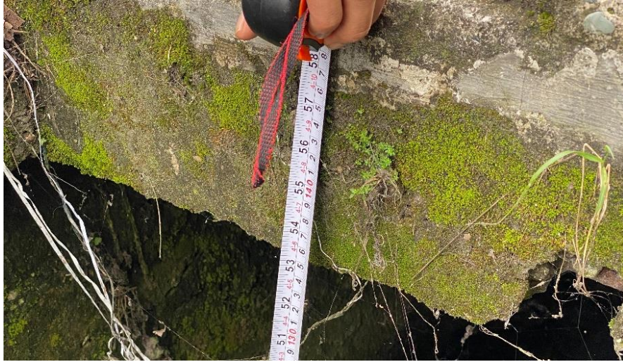
Pengukuran Drainase Eksisting Kedalaman 1,35m STA 2 + 000
