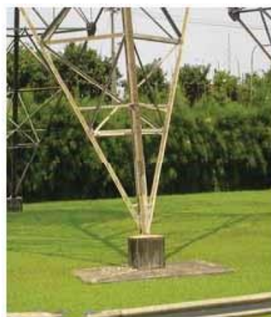
gambar 12 : Pondasi Tower (Latice) SUTET 500 kV
