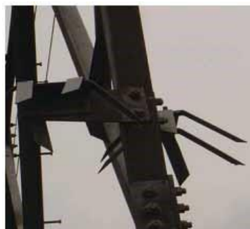
gambar 17 : Anti Climbing Ddevice (ACD)
