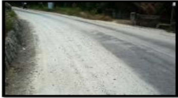
Gambar 2.18 Pelepasan Butir ( Weathering/Raveling )
