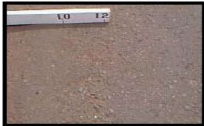
Gambar 2.14 Pengausan Agregat ( Polished Aggregate )
