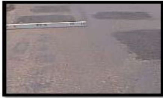
Gambar 2.13 Tambalan dan Tambalan Pada Galian Utilitas (Patching And Utility Cut Patching) (Sumber : Bina marga no. 03/MN/B/1983 )
