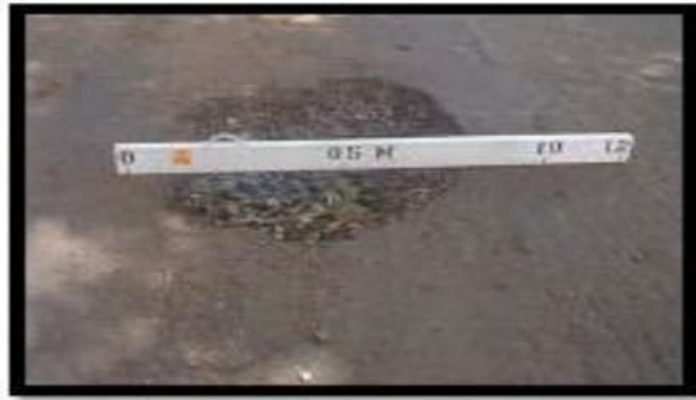
Gambar 2.15 Lubang ( Potholes )
