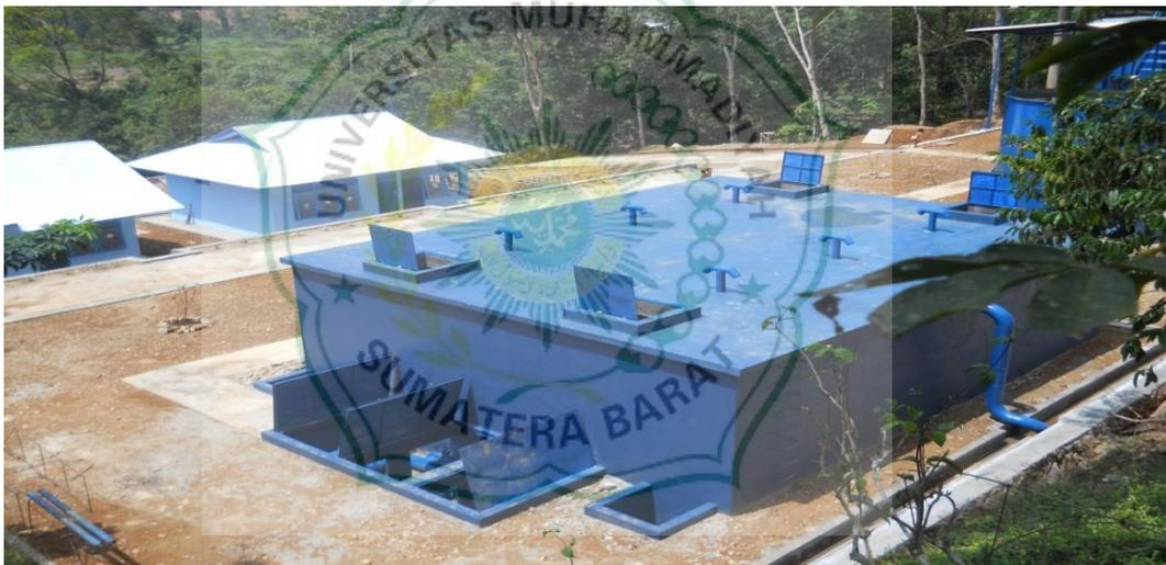
Gambar 2.4 : Bak Reservoir Kap 300 M3
