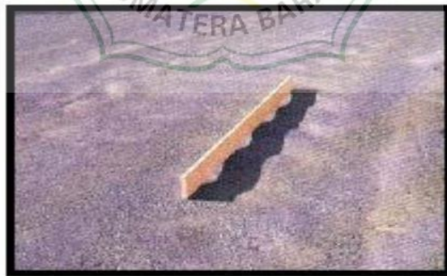
Gambar 2.4 Retak Kriting ( Corrugation Cracking ) (Sumber : Bina marga no. 03/MN/B/1983 )
