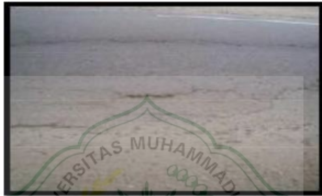
Gambar 2.7 Benjol Dan Turun ( Bumb And Sags ) (Sumber : Bina marga no. 03/MN/B/1983)
