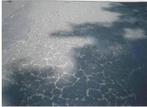
Gambar 2.19 Pelepasan Butir ( Weathering/Ravelling ) Sumber : Google (2021)
