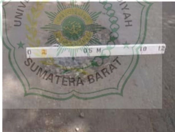
Gambar 2.13 Lubang ( Potholes )
