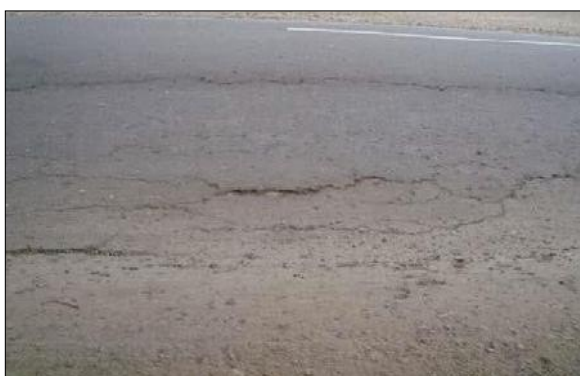
Gambar 2.4 Cekungan ( Bumps and Sags )
