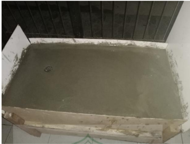
Gambar .3.2 Tungku re-heating lubang output diameter 50 mm
