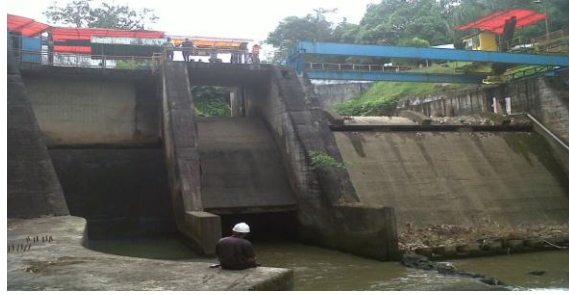
Gambar 2.13. Intake weir
